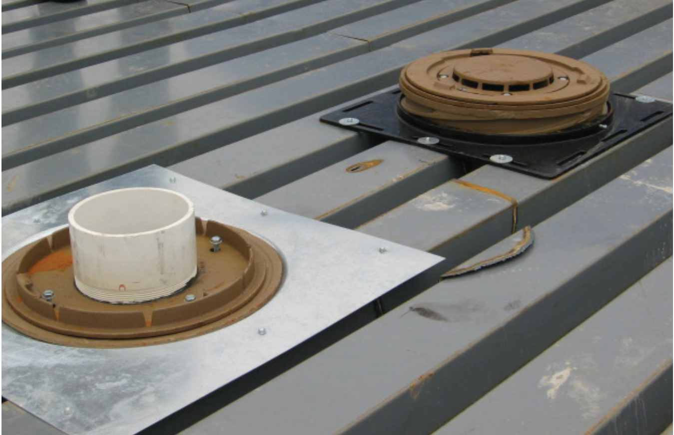
Figure # 1070 Overflow Standpipe Drain used with Figure #1005 Siphonic Roof Drain.
