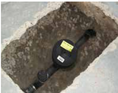
View of a Flood-Gate installed in a 4-foot deep concrete pit.
