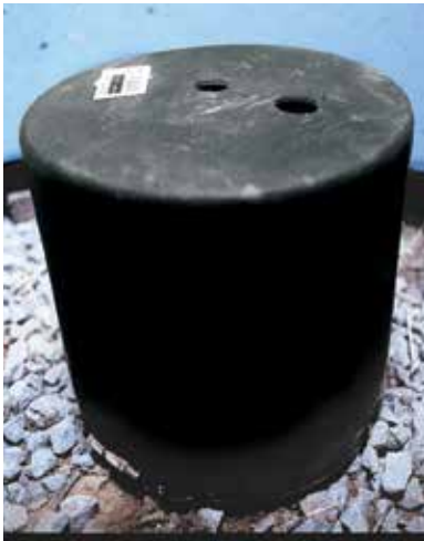
View of Flood-Gate in plastic pit with gravel ballast.
