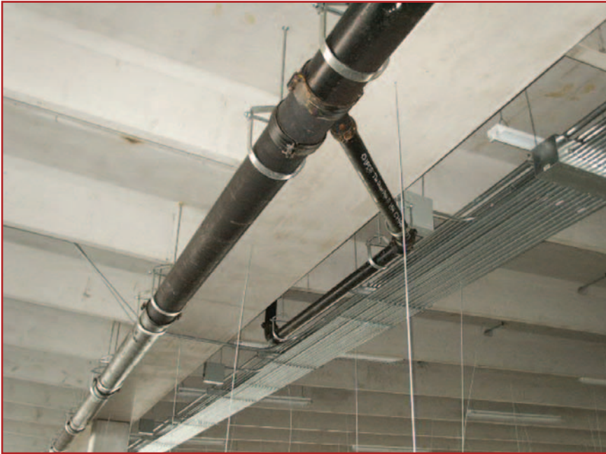
A drain tailpiece joining with a horizontal manifold.
