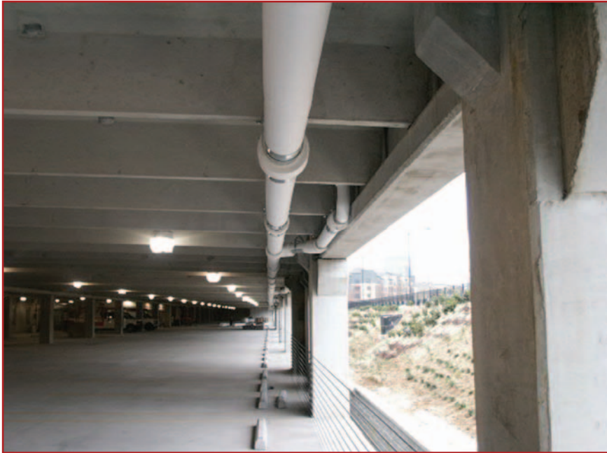
A horizontal drain manifold overhead at an IKEA in Atlanta, GA.
