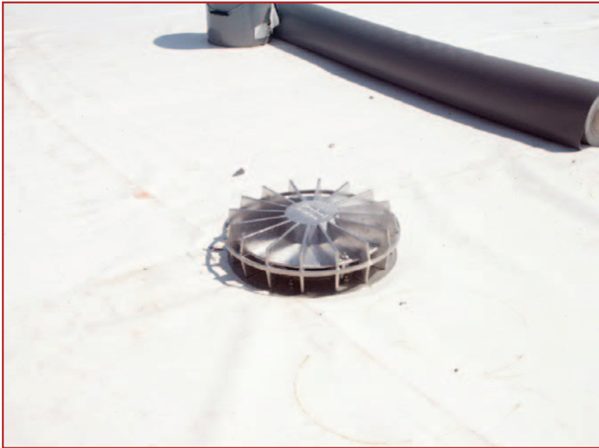
A typical baffled siphonic roof drain.
