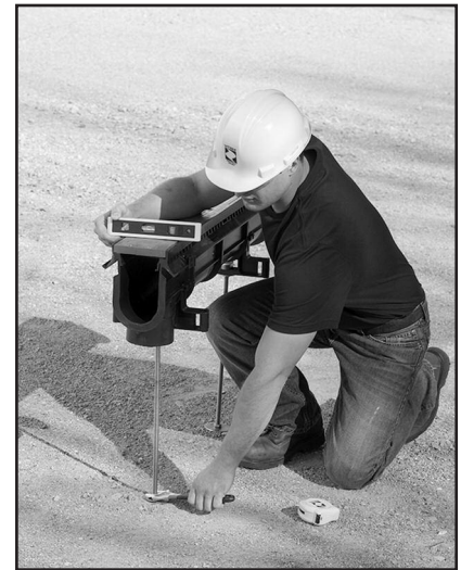
Setting adjustment nut and plate - Step 7
