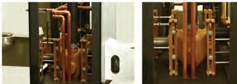
Wall chase images featuring a Fig. # 0240DY-M54 closet support installation.
