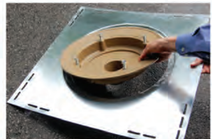
2. Place 1010 roof drain into the sump receiver deck plate.
