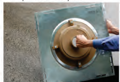
4. Place the deck plate and roof drain combination on the roof and attach the deck plate to the roof structure.
