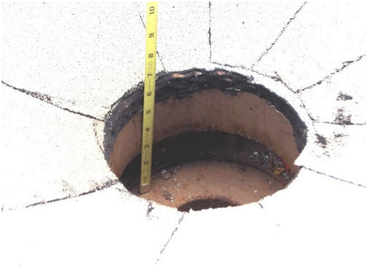
MEMBRANE CUT AT INSIDE DIAMETER OF THE SUMP CORRECTLY
