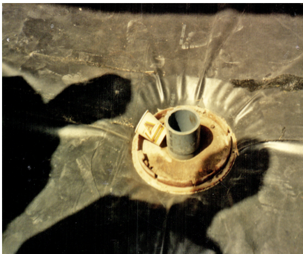
THE MEMBRANE APPEARS TO BE INSTALLED CORRECTLY WITH THE 1080 ROOF DRAIN UPON REMOVING THE COLLAR, IT WAS BUNCHED UP IN THE ROOF DRAIN SUMP
