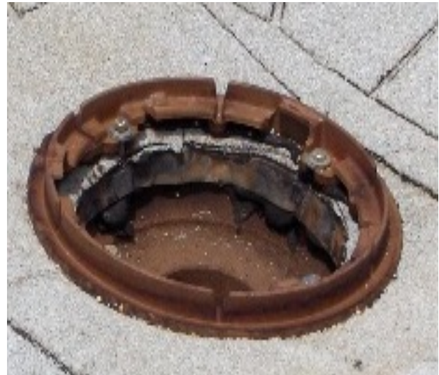
CLAMPING COLLAR INSTALLED
