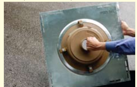
4. Place the deck plate and roof drain combination on the roof and attach the deck plate to the roof structure.
