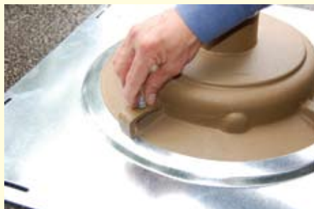
3. Bolt the 4 angled steel support brackets onto the roof drain until the deck plate is locked into place. (See -DPK Trim Kit)
