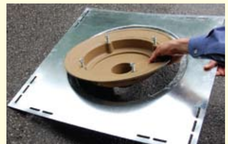
2. Place 1010 roof drain into the sump receiver deck plate
