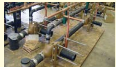
Fig. No. 0210RY-M54. Board mounted water closet with water supply lines.
